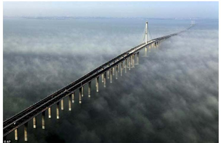
*This immense £1 billion structure is supported by more than 5,000 pillars, stretching for 24 miles along China's eastern port city of Qingdao to the offshore island Huangdao. It is an Engineering feat par excellence, becoming the largest cross-ocean bridge in the world.*
